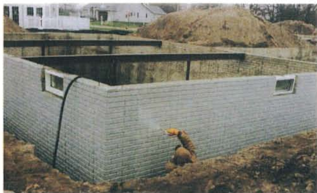
One type of high quality waterproofing is a gray, all rubber membrane. Others are black asphalt with rubber polymers added to give them flexibility.
